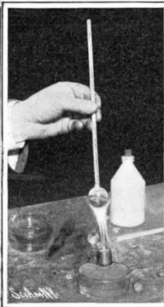
Creating a Vacuum by Boiling Mercury in the Bulb.
