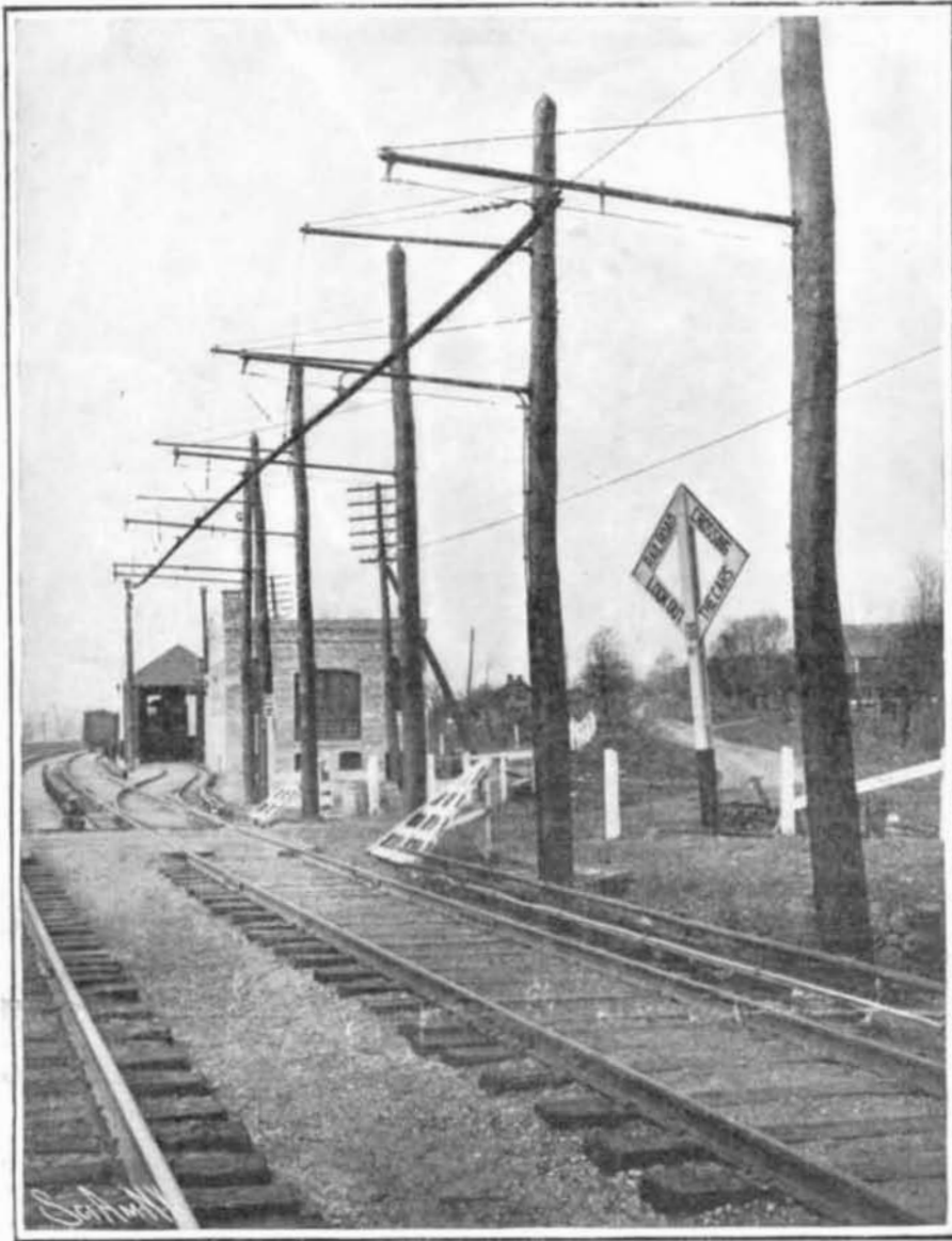
Experimental Track, Showing Third Rail ; Overhead Conductor at Crossing; and the Substation.
