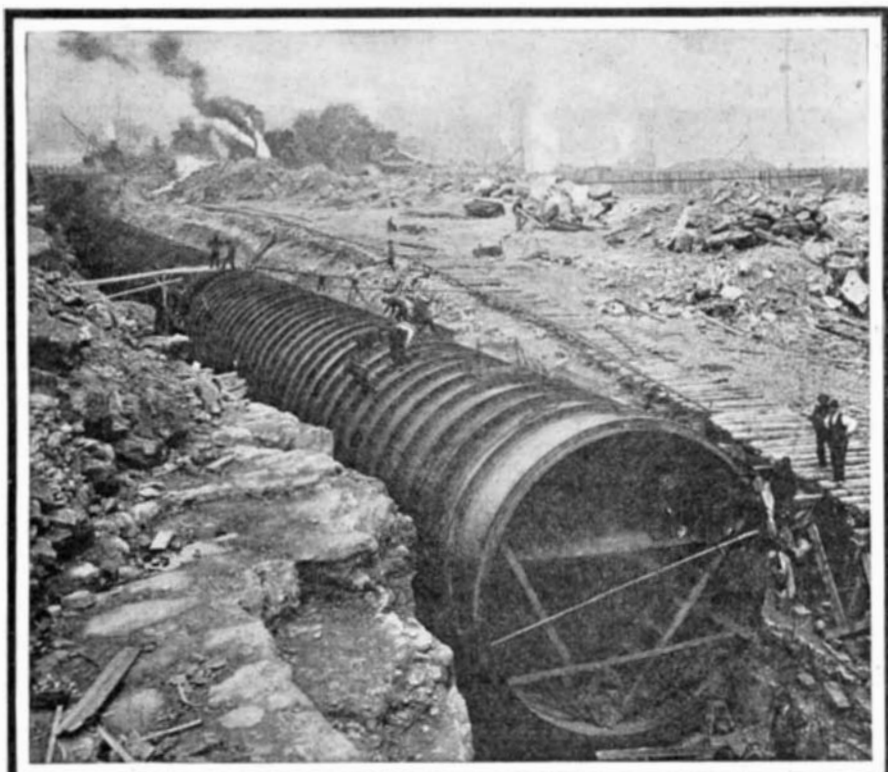
Laying One of the 18-foot Steel Flumes. These Will Everywhere be Buried From Sight.
