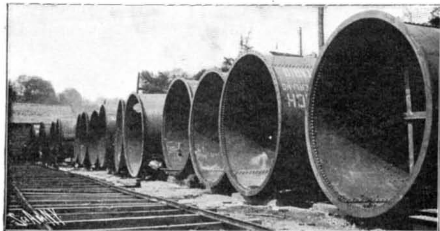
Sections of the 10-Foot Penstocks, Through Which Water is Conveyed from the Forebay, Vertically, to the Turbines at the Bottom of the Wheelpit.
