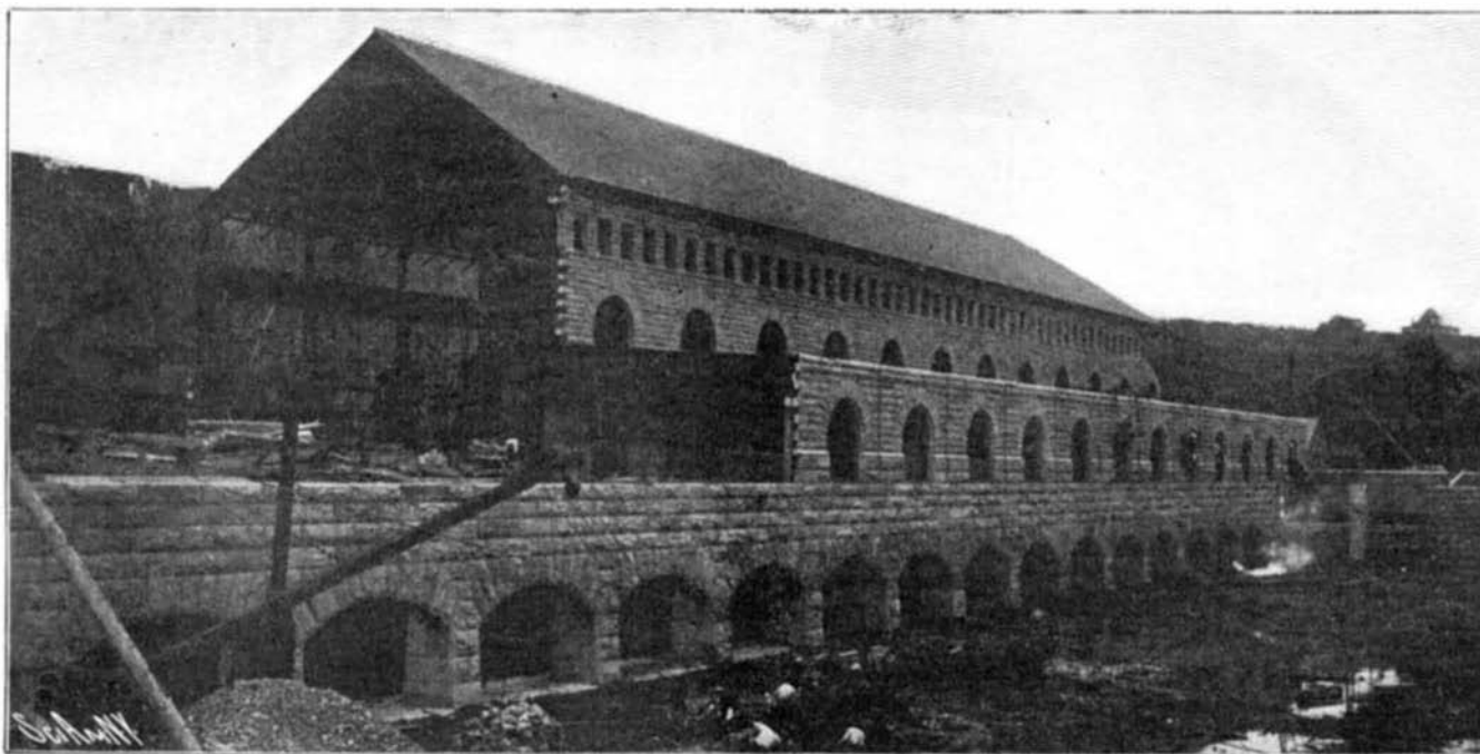
Power Station Partially Completed, Showing the Forebay, the Arched Entrances Through Which the Water Flows to the Penstocks, and the Main Generating House to Contain Eleven 10,000-Horse-Power Generators.
