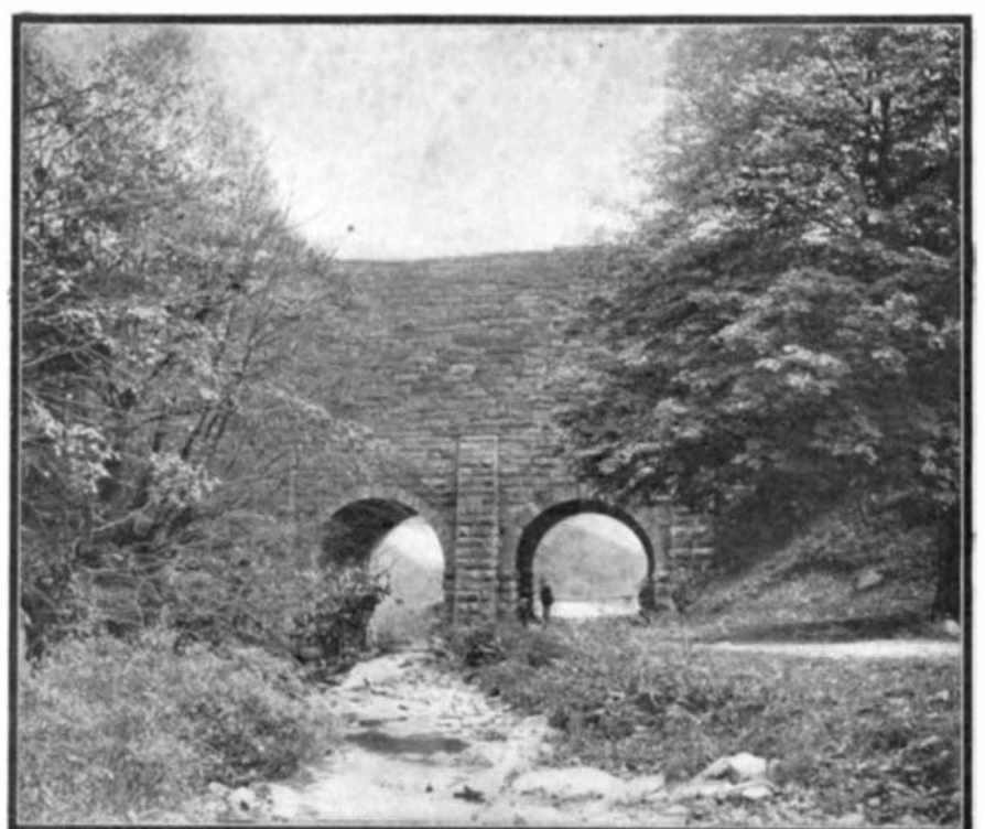
MASSIVE STONE CULVERT, RECENTLY DESTROYED. ERECTED IN 1848 ON THE LINE OF THE NEW PORTAGE RAILROAD.
