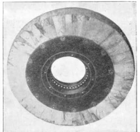
Fig. 4.—Wheel Formed of Wood Segments, Showing Ball Bearing in Hub.
