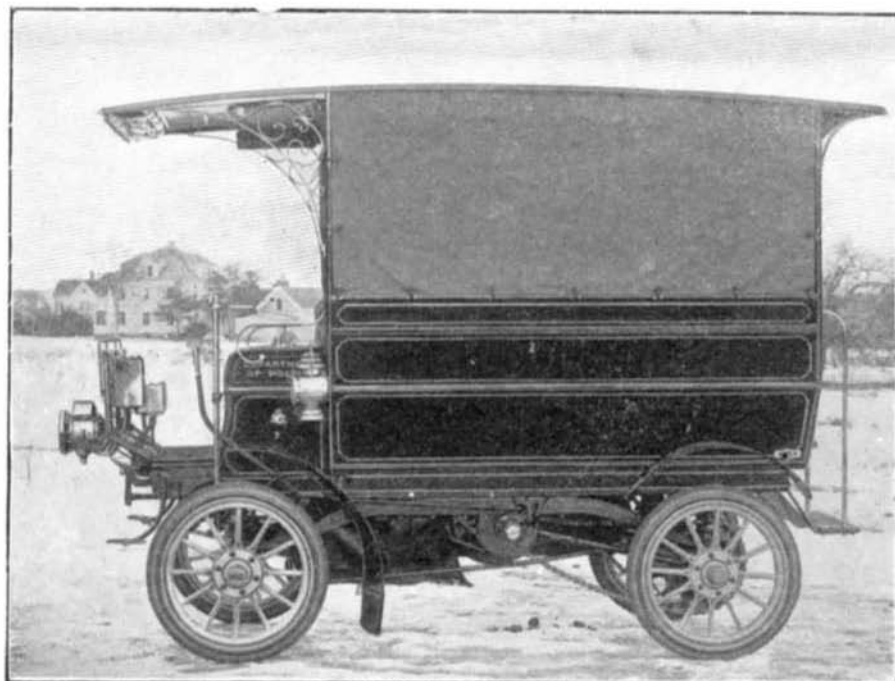
Knox Patrol Wagon Propelled by 16-Horse-Power Horizontal Air-Cooled Motor.
