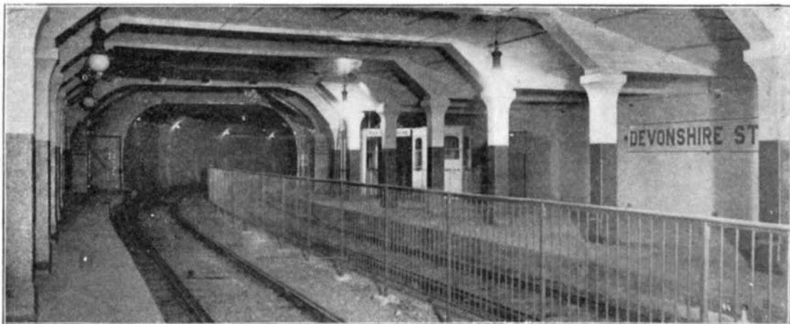
Devonshire Street Station, Showing Method of Interior Finish.
