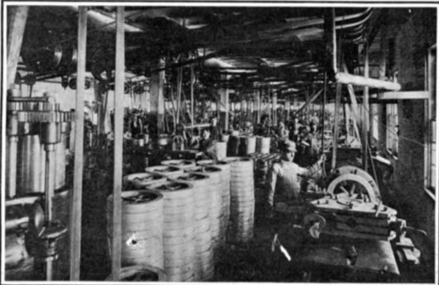
Main Machine Shop at Reo Works, Where 5,500 Parts Are Made Daily.
