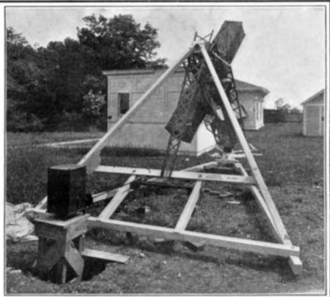
One of the Polar Axes with Camera Mounted and Temporarily Covered for Testing.
