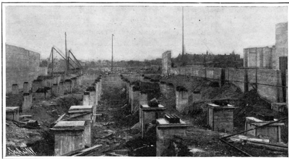
Columns Supporting the Interior Structure.
