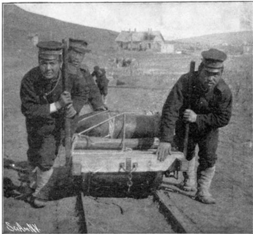
The mortars, their mounts, and the materials for the concrete emplacements, were all brought to the site of the batteries over a narrow-gauge road, which was under fire for two months.
