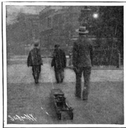
Testing a Pavement.
