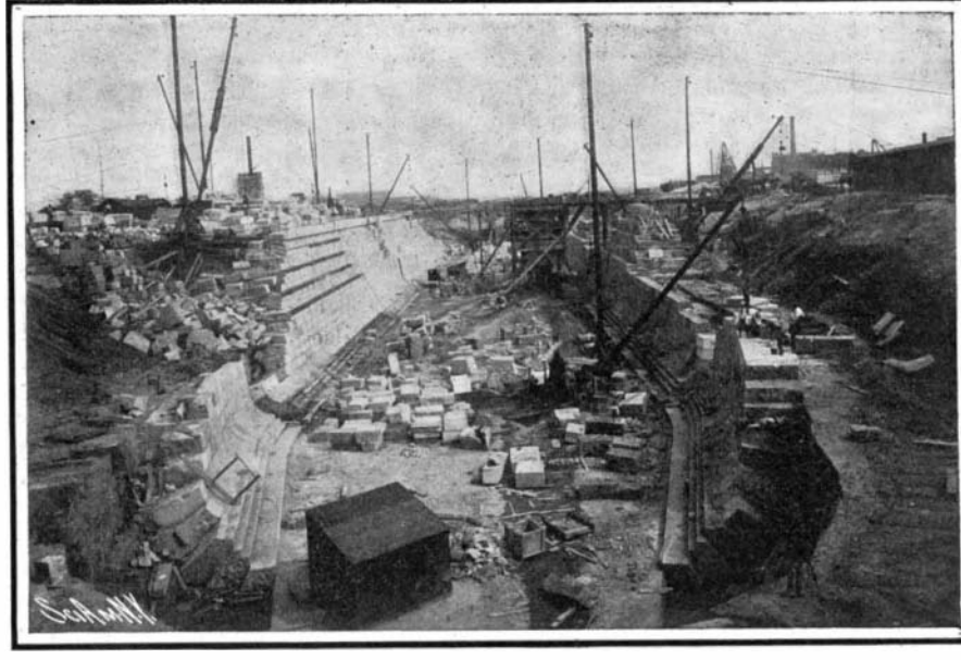
Looking Toward Dock Entrance.
