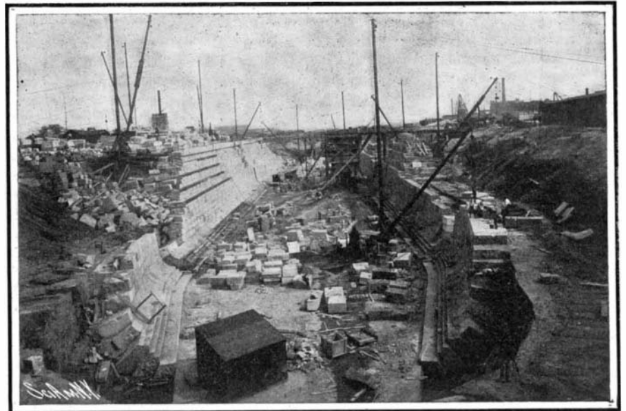
Looking Toward Dock Entrance.
