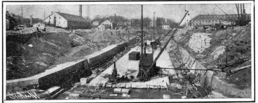
View Looking from the Dock Bulkhead.
