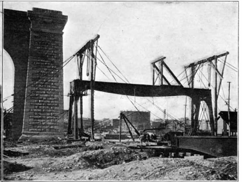
Constructing the Electric Gantry Crane for Erecting Blackwell's Island Span.
