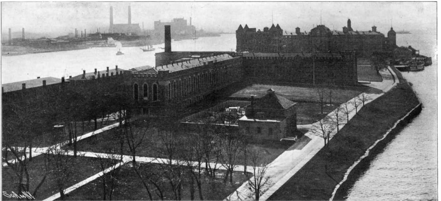
View Looking South From the Top of One of the Island Piers.
