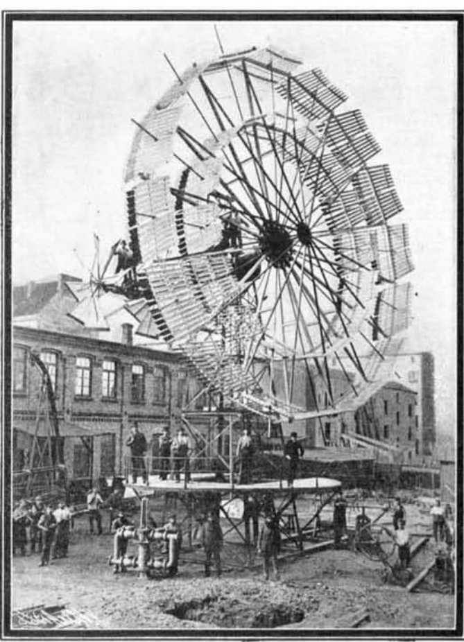
An 18-Horse-Power Wheel, 40 Feet in Diameter.
