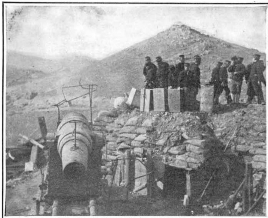
Photos. by Edwin Emerson, Jr. Seacoast Mortar, Protected by Sandbag Emplacement.
