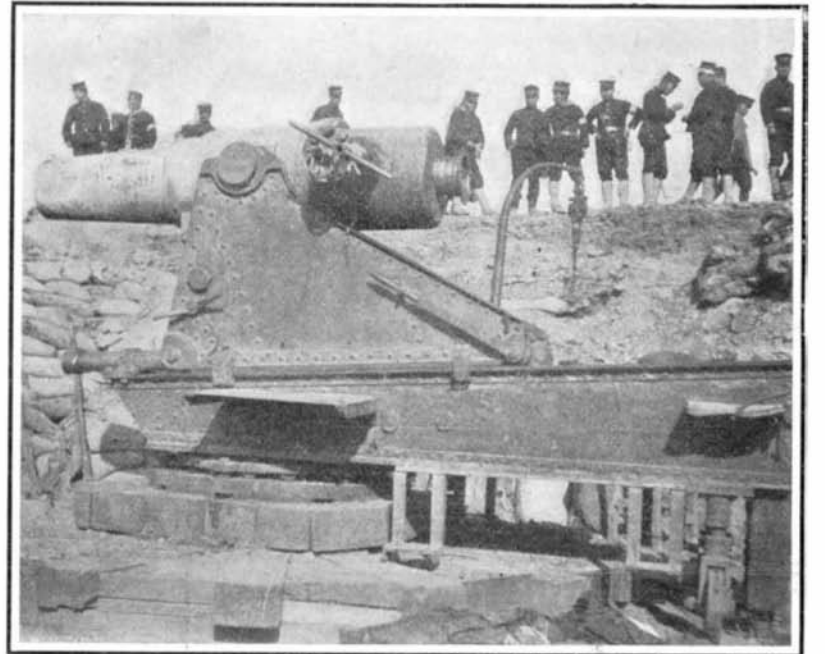
Heavy Mortar on an Improvised Foundation.
