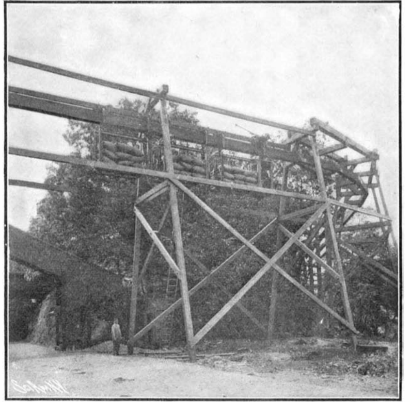
From the Storehouse, the Telpher Train Crosses the Road, Rounds the Curve, Travels along the Bank of the River, then Crosses the River upon a Steel Bridge and Enters the Mill.
