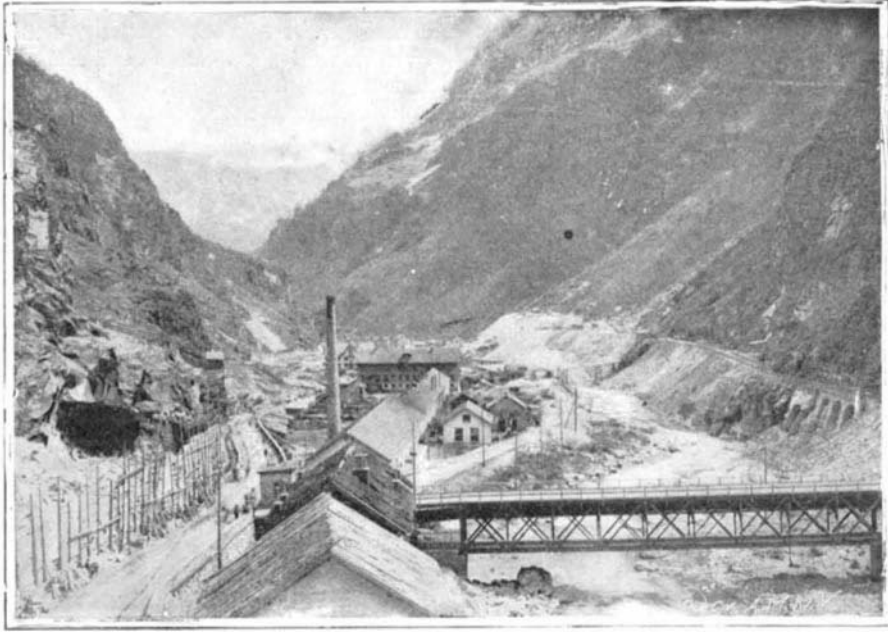
Upper Power House. Iron Bridge Across the Diveria for the Flume. To the Left, a Small Tunnel Leading to the Main Tunnel.
