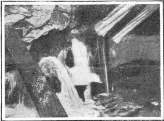
Springs Gushing from Tunnel Walls.
