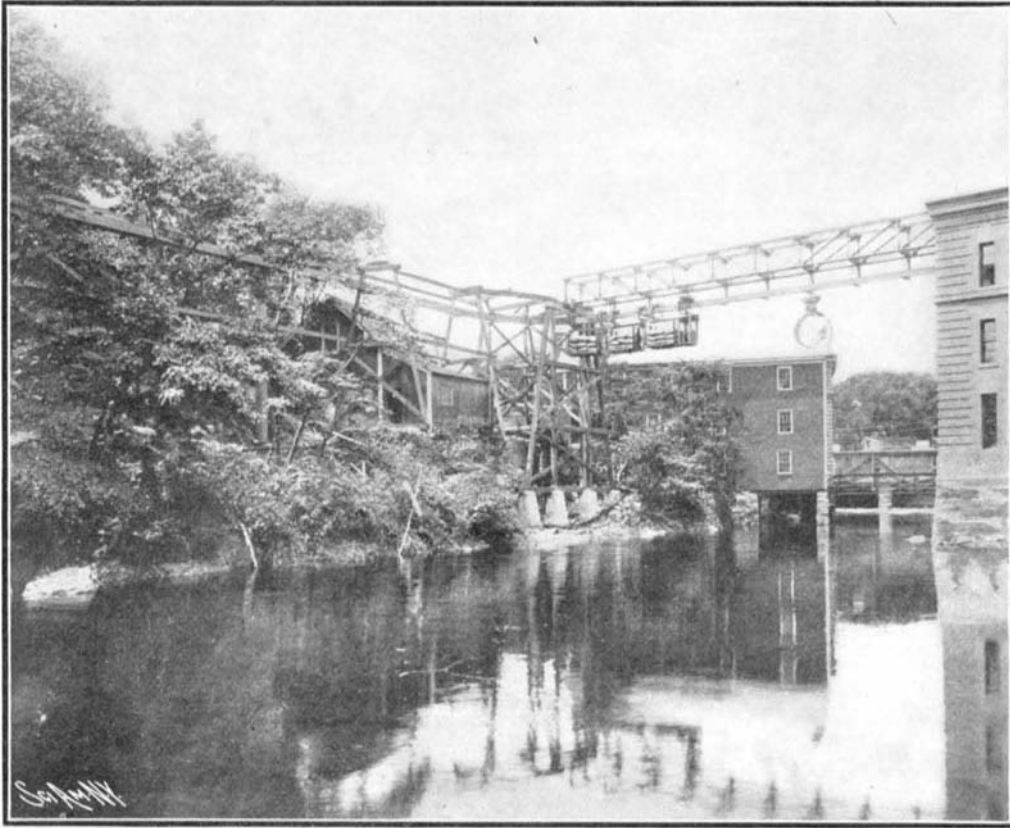
The Concrete Foundations for the Supports of the Steel Bridge Which Spans the River. Telpher with Full Load about to Pass around the Curve.
