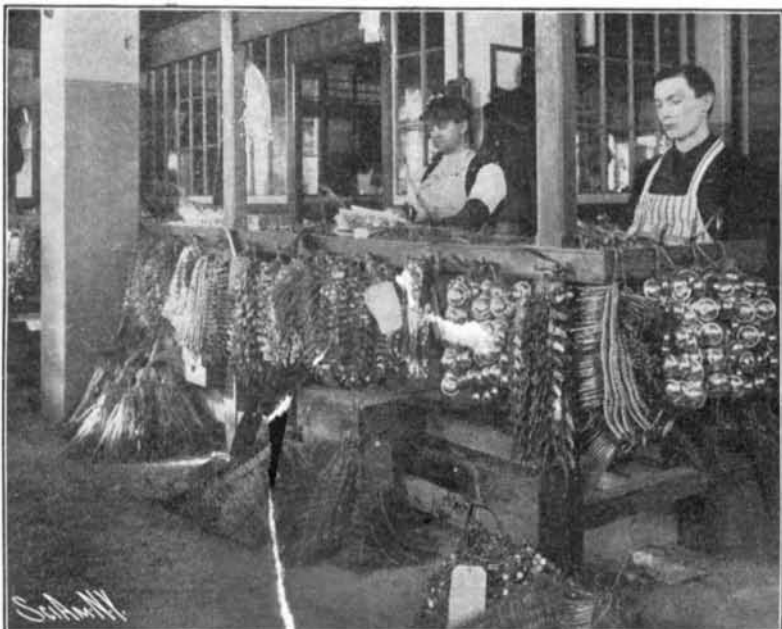
Wiring Articles for Plating.
