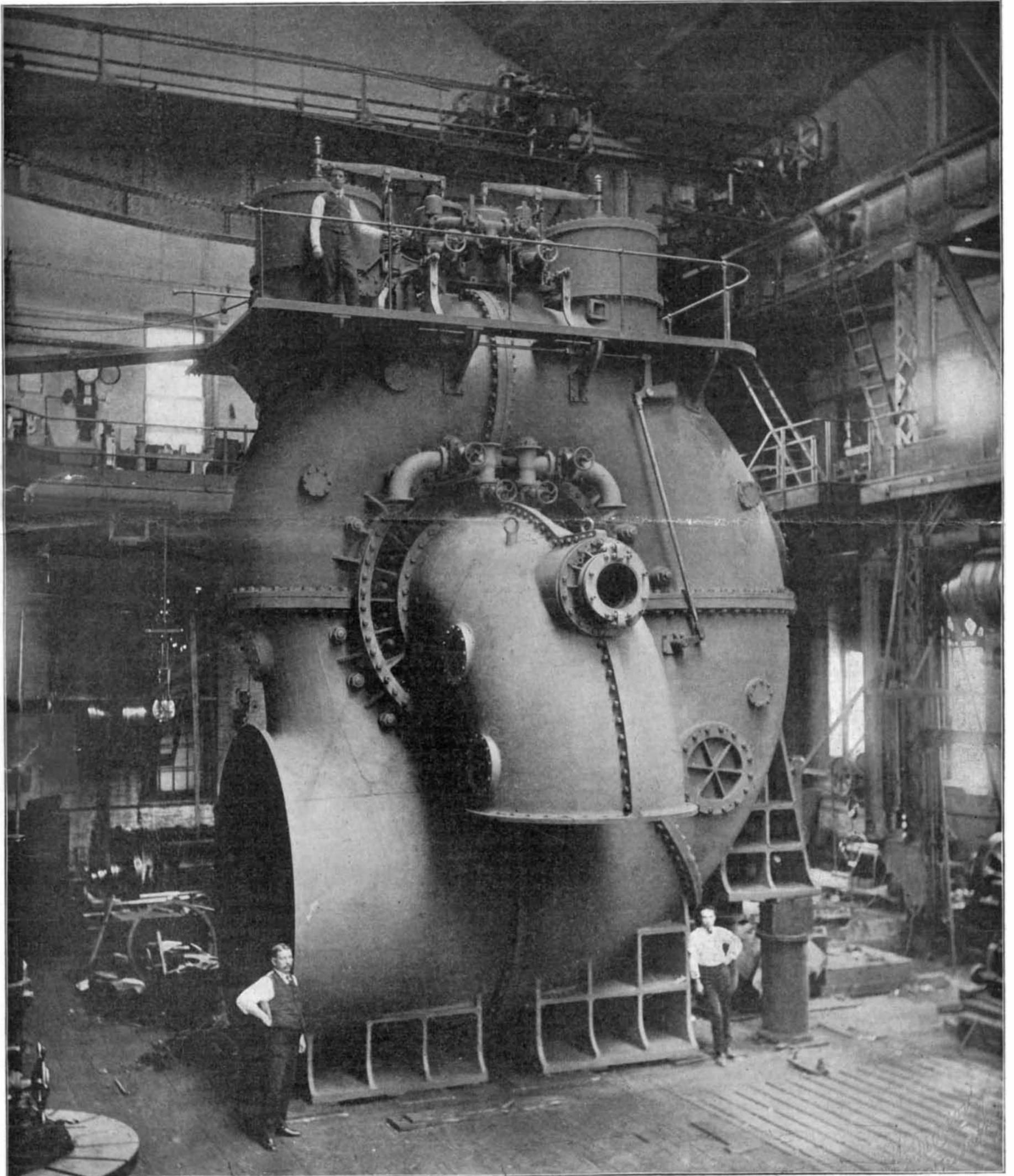
**Weight, 364,000 pounds. Height, 30 feet. Weight of Wheel, 5 tons. Weight of 22-inch Shaft, 10 tons. Intake, 10 feet diameter. Amount of water passing through per minute, 400,000 gallons. Built for the Shawinigan Power Station, Canada.**
