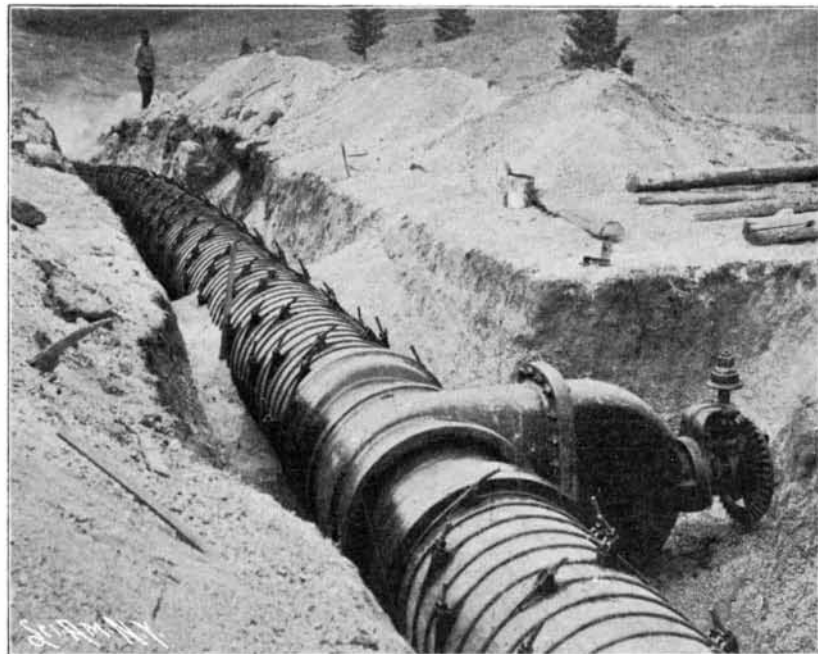
Two-foot Domestic Water Service Redwood Stave Pipe Showing Two-foot Gate.
