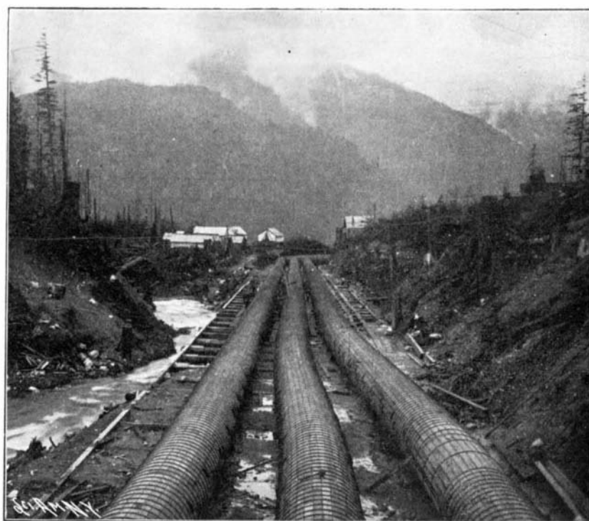
Three 54-inch Redwood Stave Pipes Used for Power Purposes.
