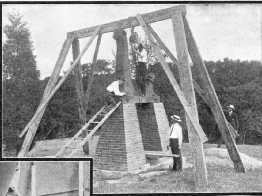
Lowering the Axis Support on the Piers.
