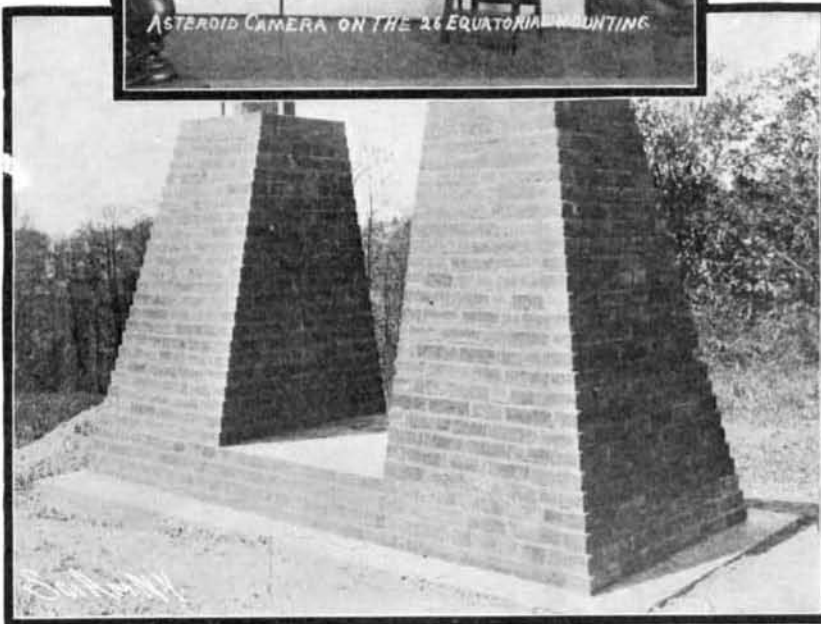
The Masonry Piers.
