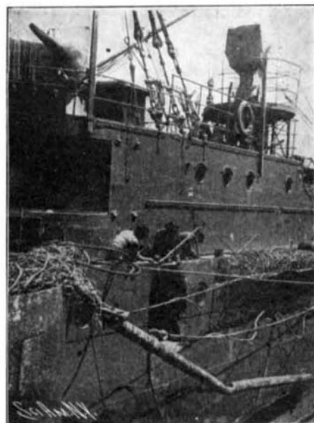
Hole Made by Large Shell Just Below Main Deck.
