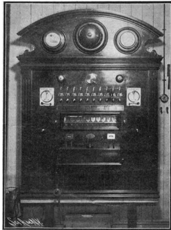
Fig. 2.—Fire Alarm Switchboard.
