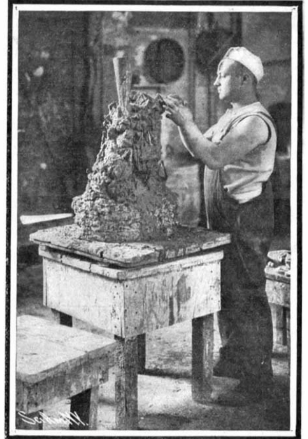
Putting on Channels, Gates, and Cores.
