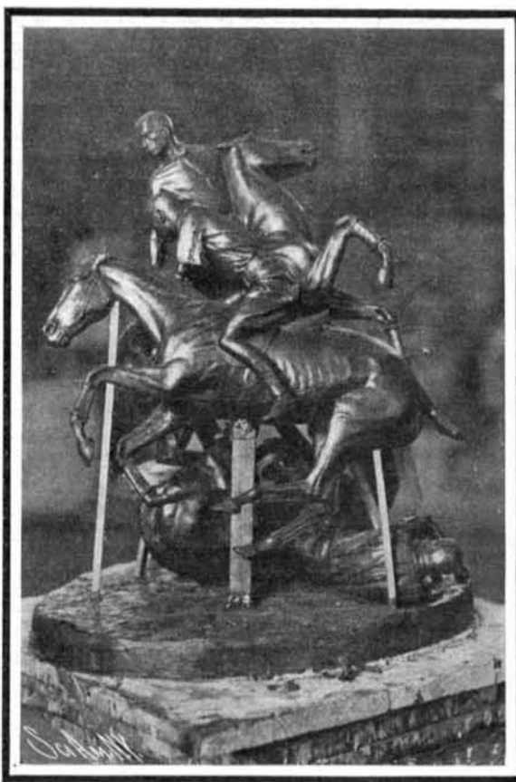
Completely Assembled Wax Positive or Pattern.
