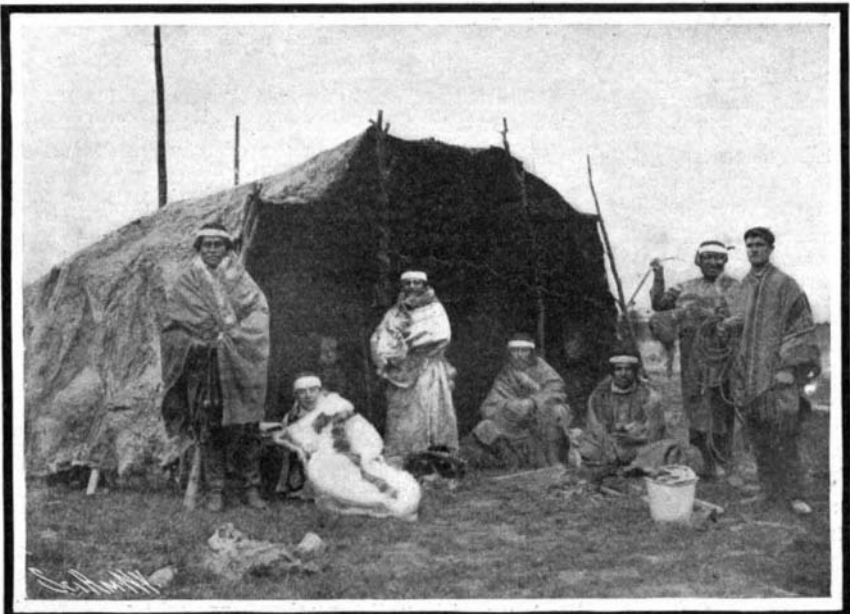
Patagonians in Front of Native Hut of Pole Framing Covered with Hide.
