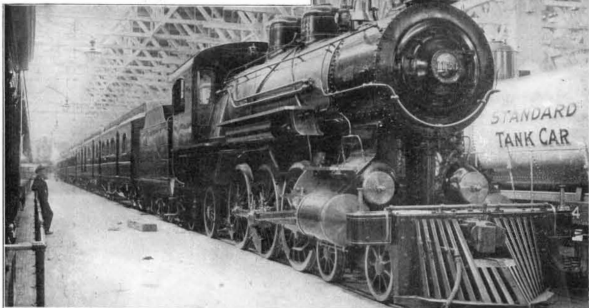
Cylinders, 20 x 26 inches. Driving wheels, 69 inches diameter. Heating surface, 2,930 square feet. Working pressure, 200 pounds. Weight of engine, 183,200 pounds.
