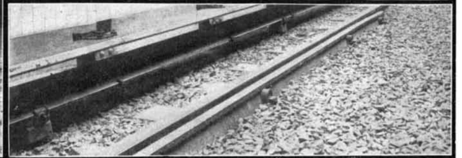
Section of Third Rail with Covering Board in Place
