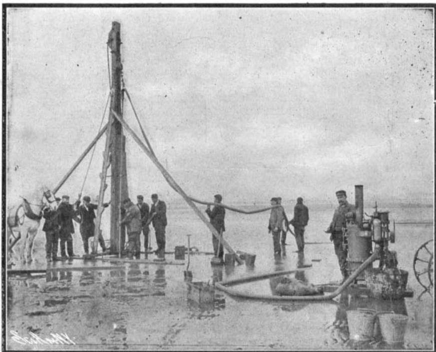
A FIRE-ENGINE USED IN PILE DRIVING.
