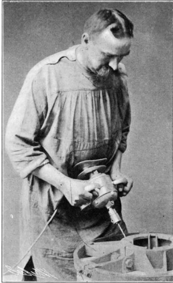
HOW THE ELECTRIC DRILL IS MANIPULATED.
