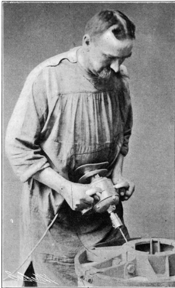
HOW THE ELECTRIC DRILL IS MANIPULATED.
