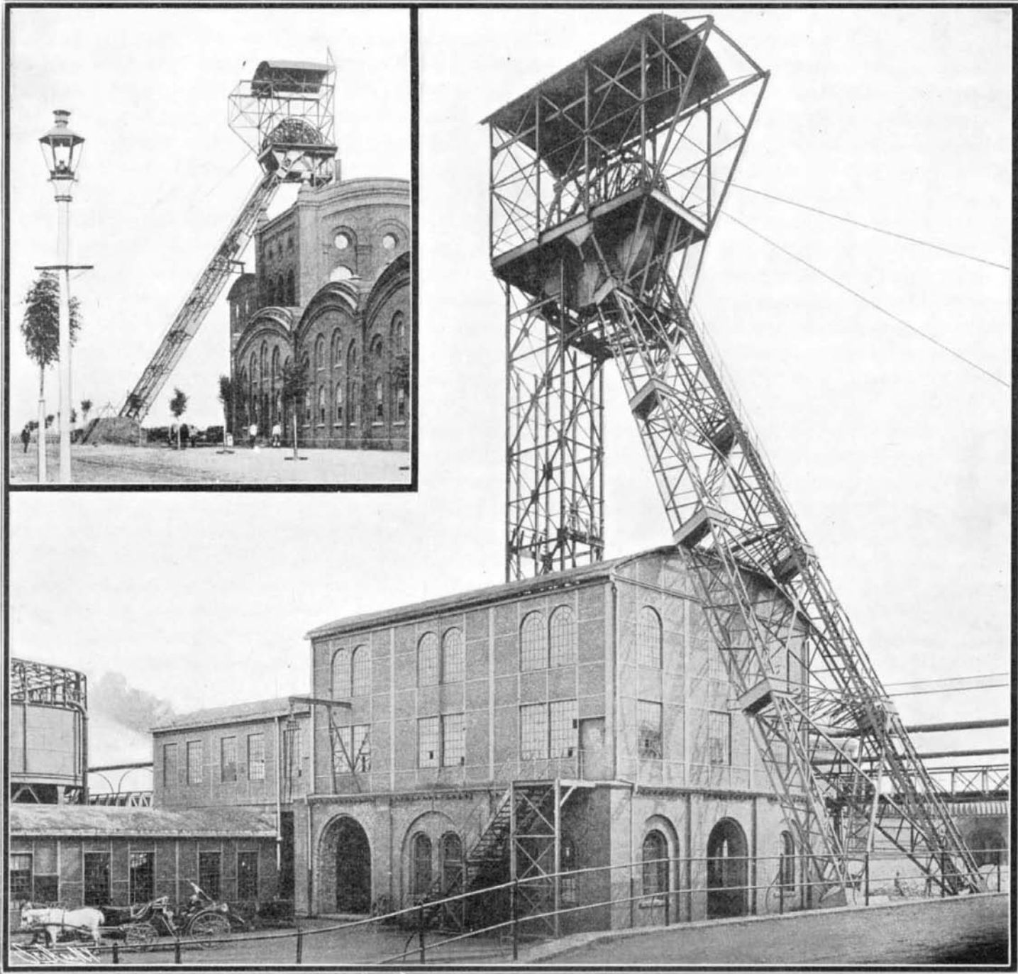
THE SHAFT OF THE RHEINPREUSSEN MINE.
