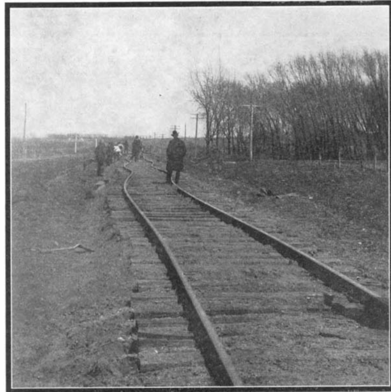
BAD CASE OF WARPED RAILROAD TRACK.
