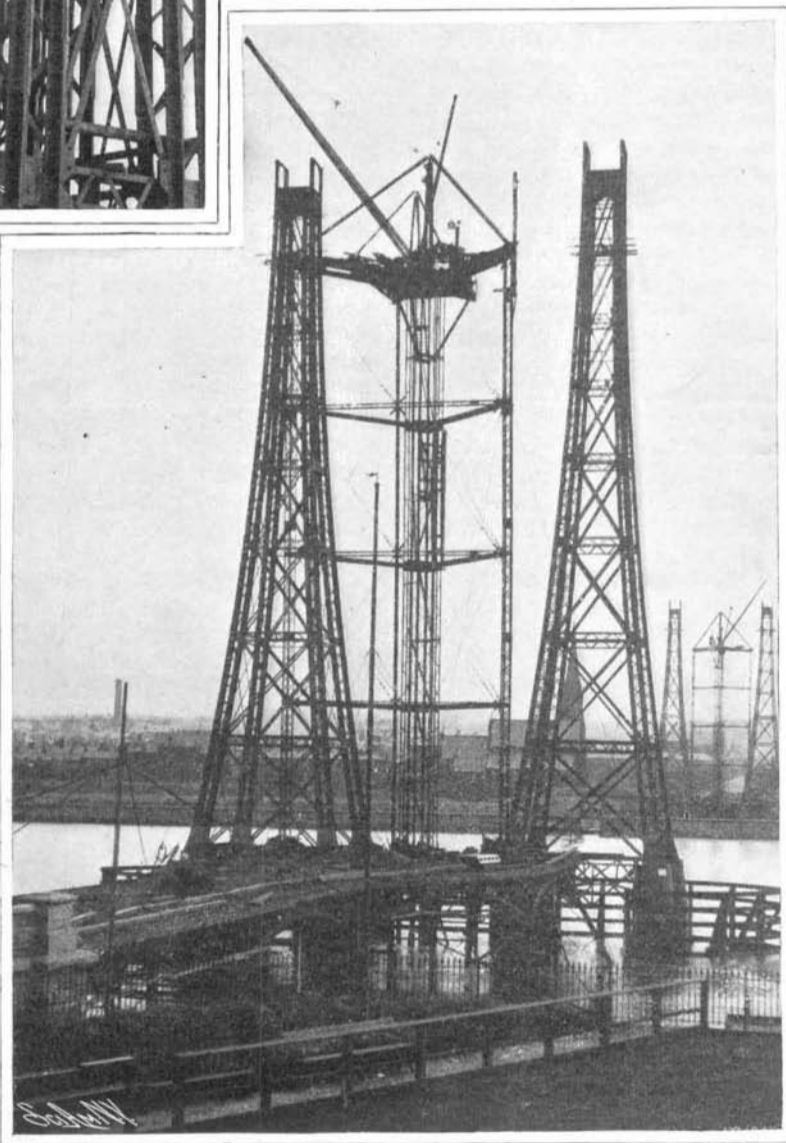
The Towers in Course of Construction. The Top of a Tower. General View of Transporter Bridge Towers on Both Banks.
