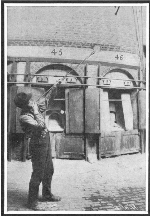
Blowing a Glass Blank
