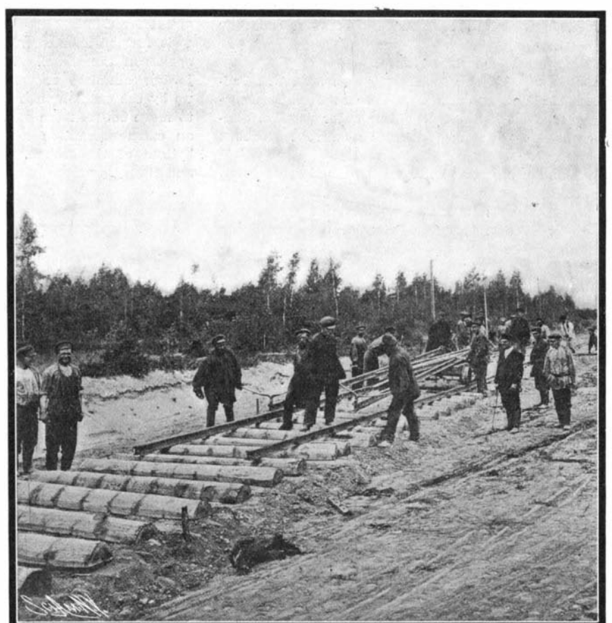
Track Laying on the Trans-Siberian Railroad; Note the Cheap, Half-Round Ties.
