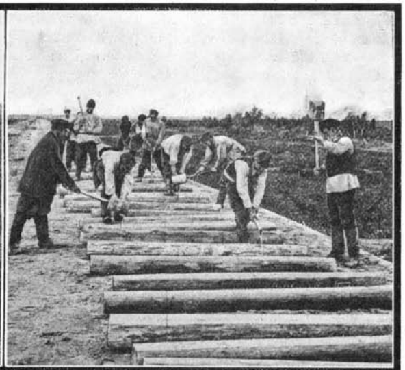
Grooving the Ties for Rails.
