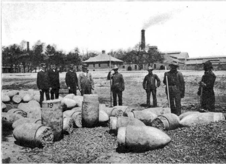
Concrete Points for Long, 17-inch Diameter Piles. Engineers' School, Washington Barracks, D. C.
