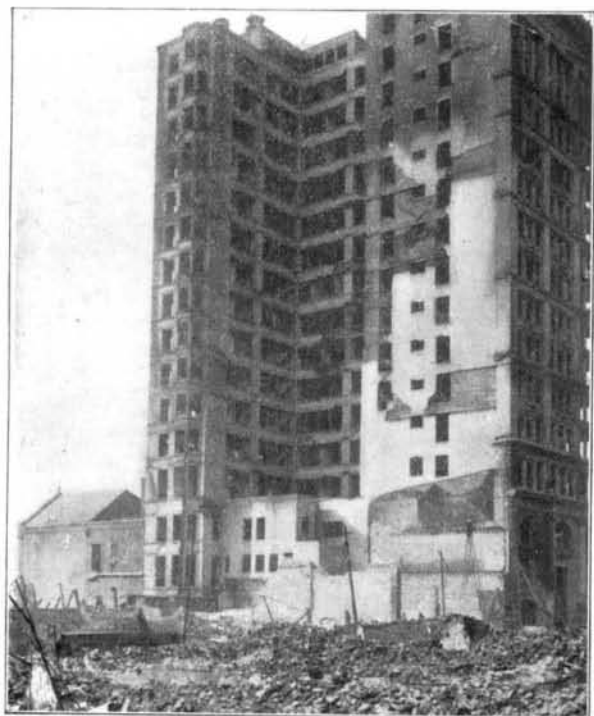
East Side of Continental Trust Building, Showing How Brick Facing was Stripped off by Fire.
