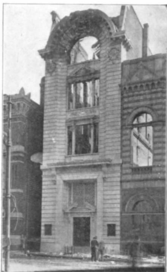
The Farmers' National Bank Building. The Three Upper Floors (Non-Fireproofed) Burned Out. The First Story (Fireproofed) was Unharmed, Not Even the Glass of Front Door Being Broken.
