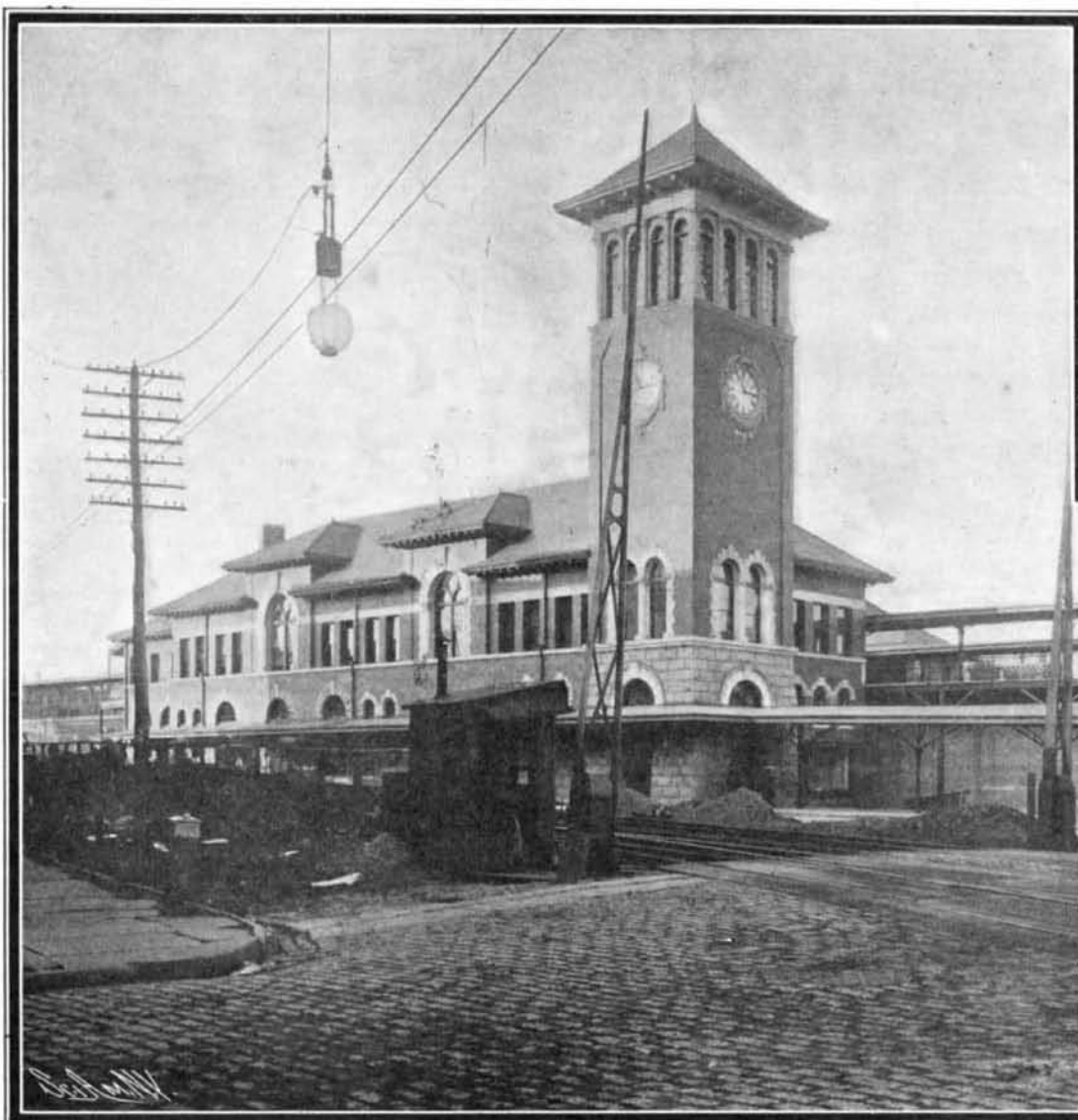
General View of New Passenger Station Showing Old Tracks in Foreground and the New Tracks Elevated. RECONSTRUCTION OF THE LACKAWANNA RAILROAD TRACKS THROUGH NEWARK.
