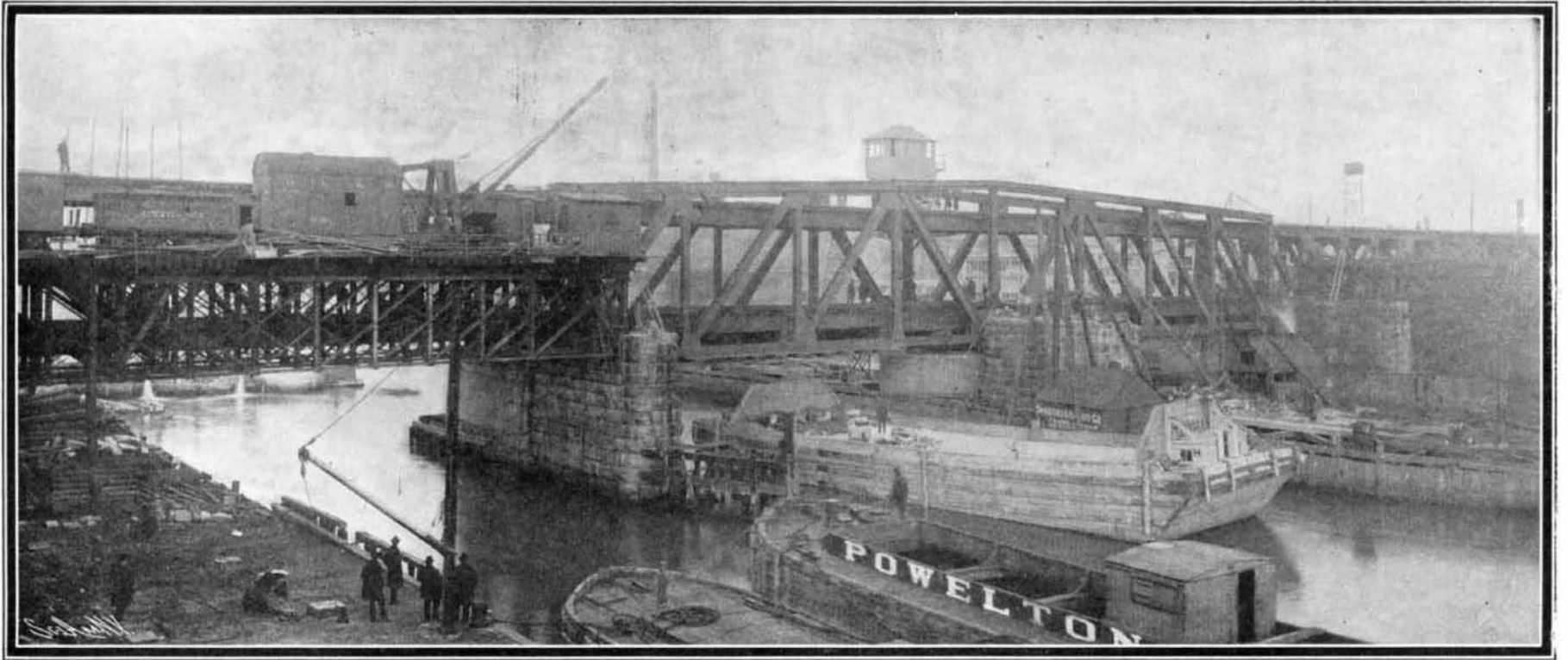
Old approaches and old draw pier in foreground. Double-Decked Draw-Span, Moved from Old to New Pier on Sunday, December 20.
