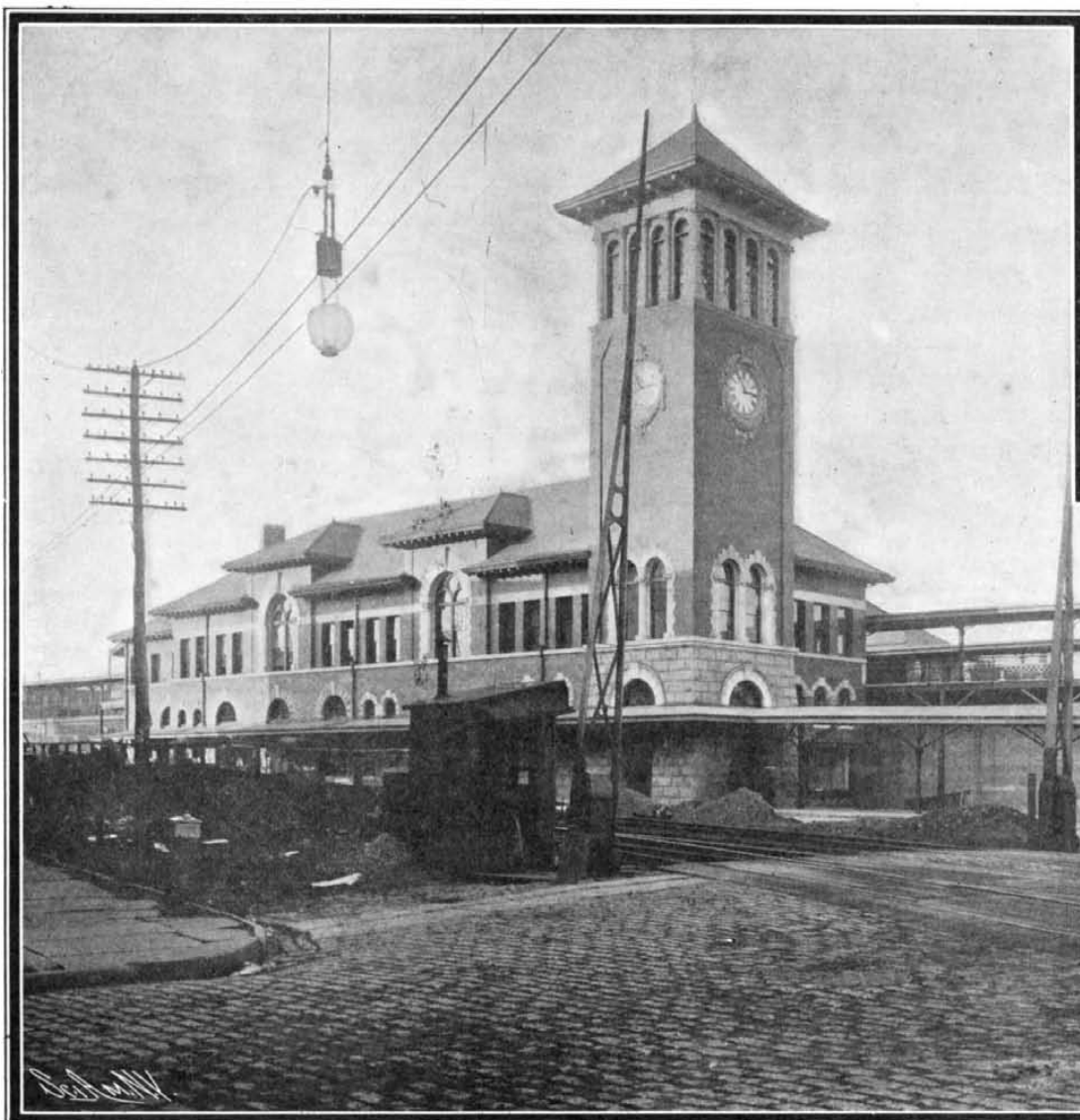
General View of New Passenger Station Showing Old Tracks in Foreground and the New Tracks Elevated. RECONSTRUCTION OF THE LACKAWANNA RAILROAD TRACKS THROUGH NEWARK.
