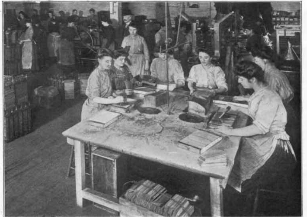
Fig. 4.—Gluing the Leads in Their Casings
