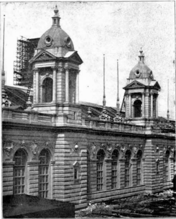
Finished Portion of Machinery Palace.
