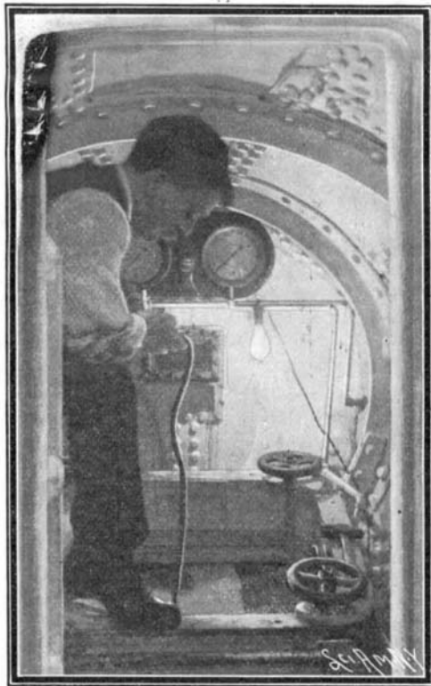
Paying Out Diver's Cable Through Diving Compartment Door.
