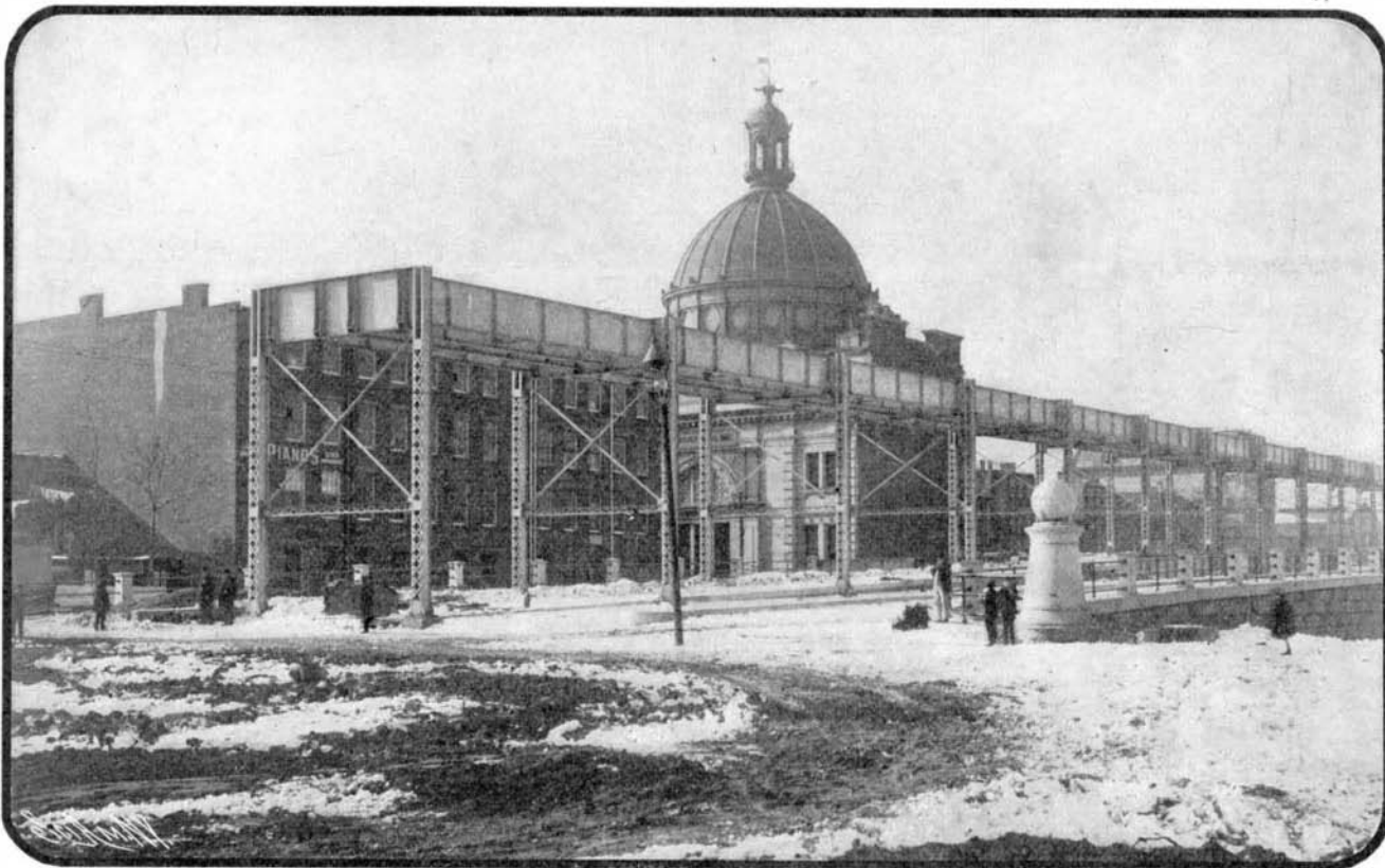
Entrance of Brooklyn Approach, Showing the Elevated Structure.
