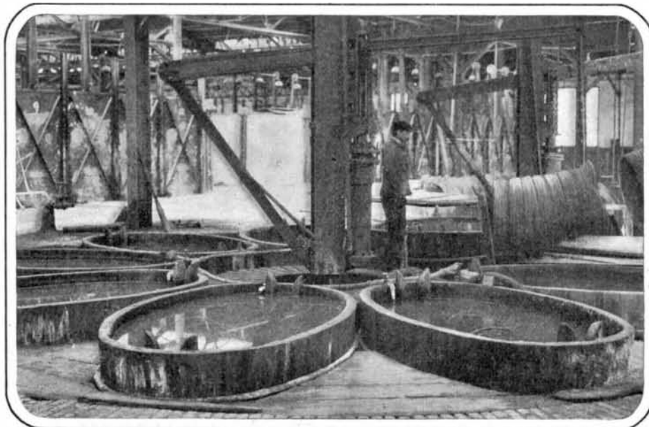
Vats of Dilute Sulphuric Acid in Which Wire is Cleaned Preparatory to Wire-Drawing.
