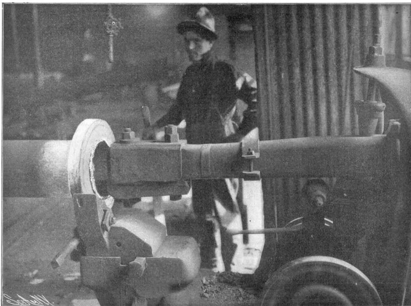
AUTOMATIC HAMMER WELDING FLANGE ON PIPE.
