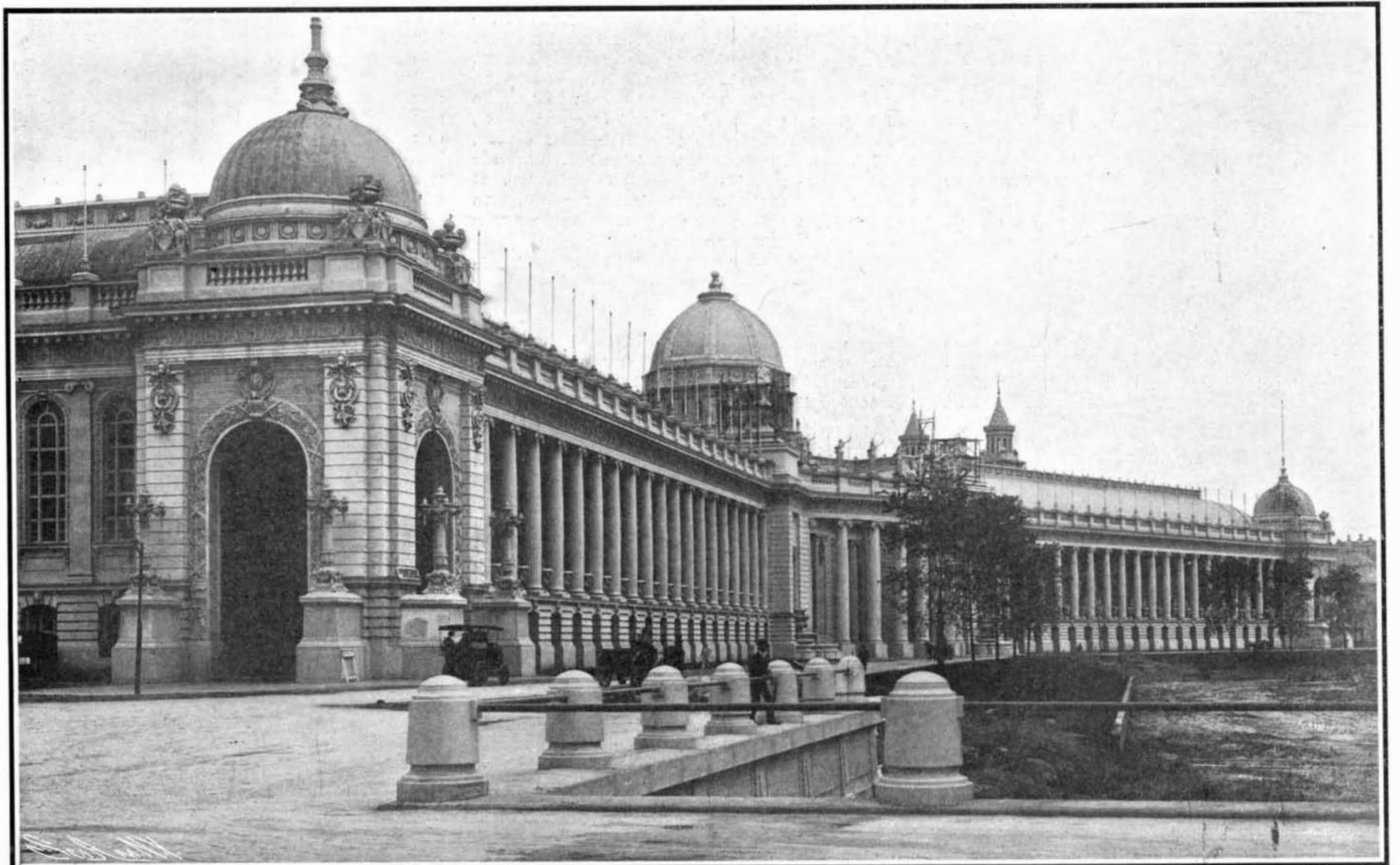
An Ionic Colonnade Veneered with Staff. STAFF—ITS USE AND TREATMENT AT THE ST. LOUIS EXPOSITION.
