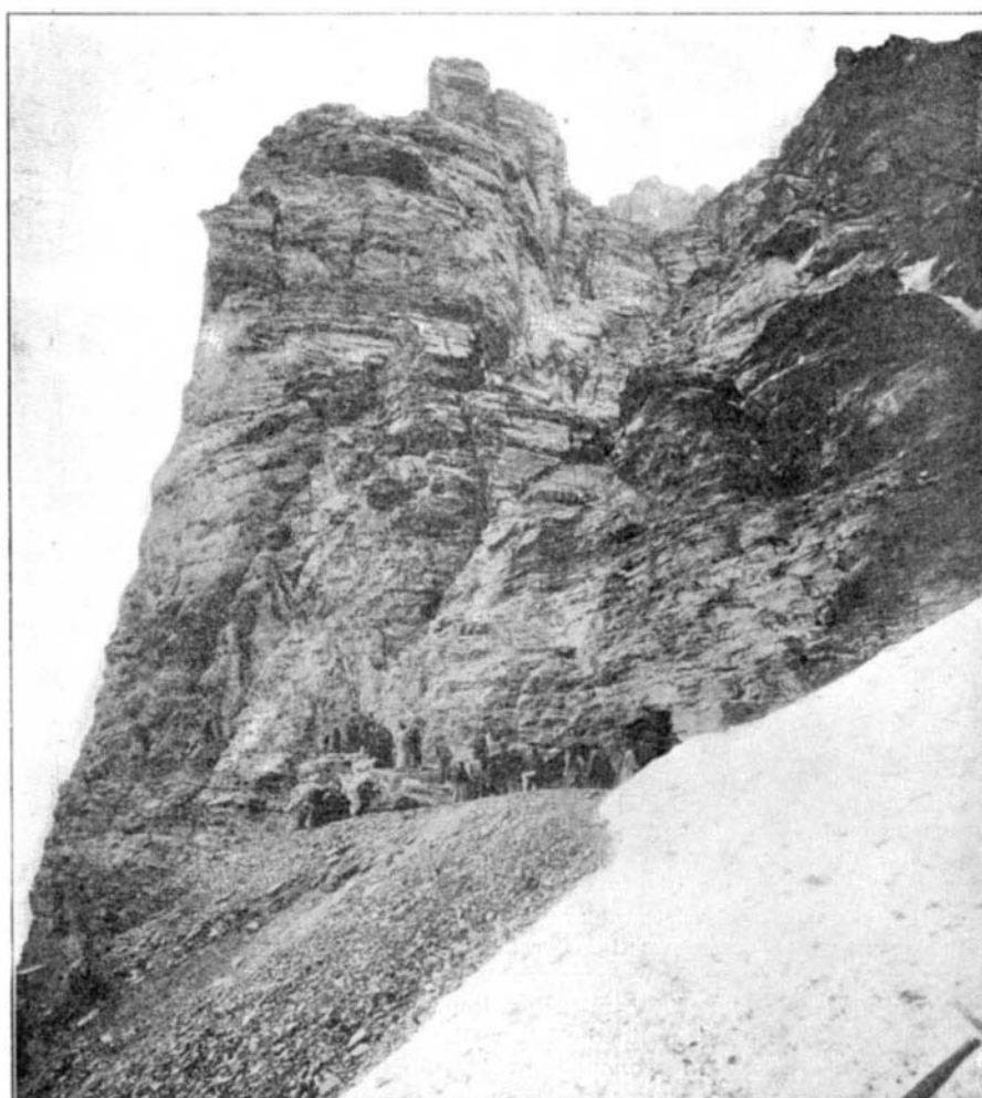
The Rothstock Station-Tunnel. Altitude 8,270 Feet. A Gallery Has Been Blasted Out of the Rock in Order that the Passengers May View the Landscape.
